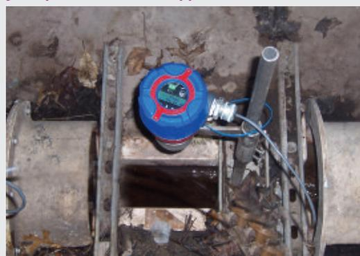
**Echotel® Model 355 Non-Contact Ultrasonic Two-Wire Transmitter for Level, Volume, or Open Channel Flow**
